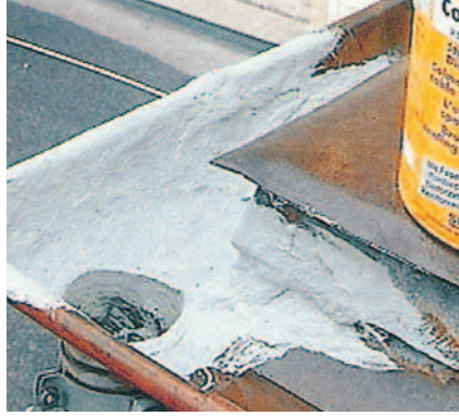
Repair gutters permanently, simply by brushing on.
