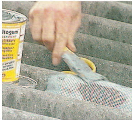
First cover large cracks with reinforcement – then apply Coltogum Water-Stop.
